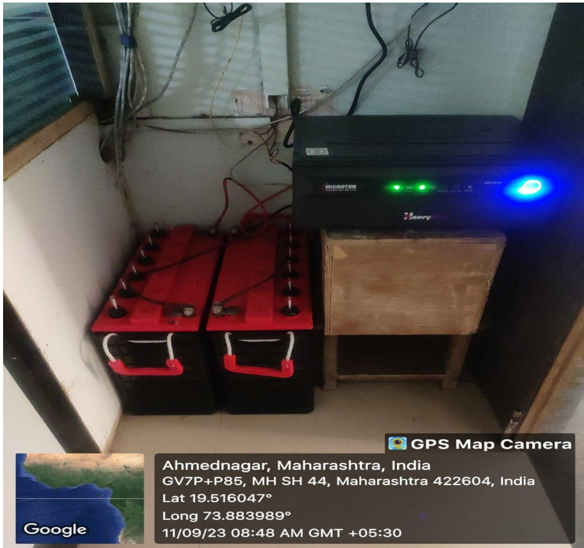
Uninterrupted Power Supply
