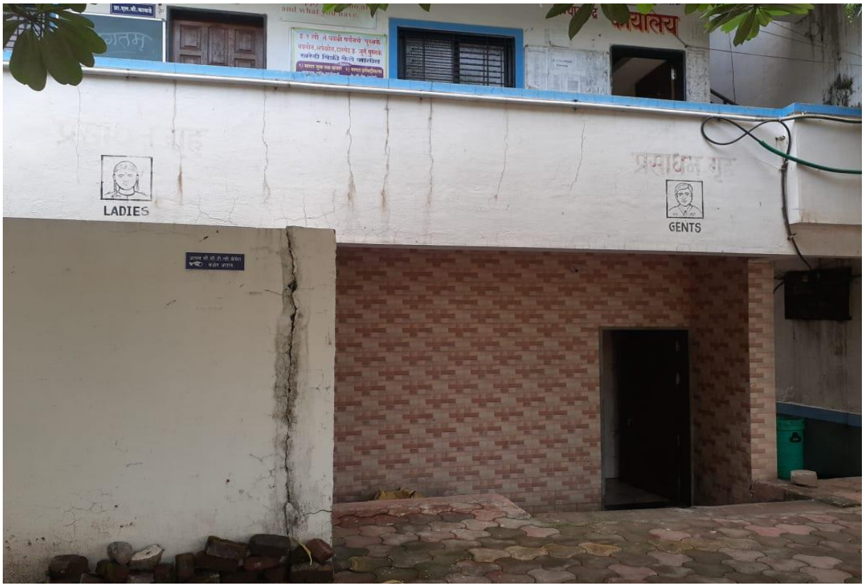
Toilet Blocks for Ladies & Gents
